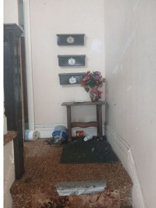
Figure 15. Vestibule with three wall mailboxes (site photo 76)
