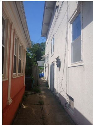
Figure 3. Stucco side wall and side passage (site photo 78)
