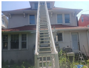
Figure 1. Rear elevation, exterior stair, upper dormer (site photo 82)
