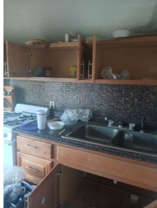
Figure 10. Kitchen two (site photo 63)
