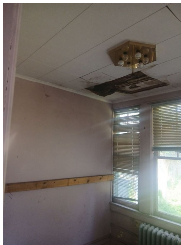
Figure 8. Ceiling opening around light fixture, radiator (site photo 19)
