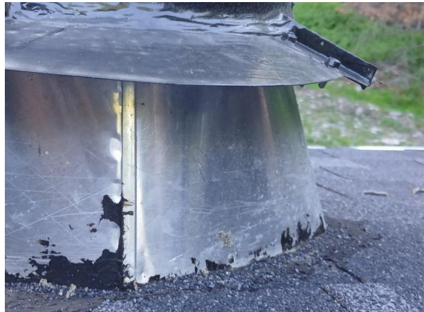
Plate 2 Flashing seam faces up the slope
