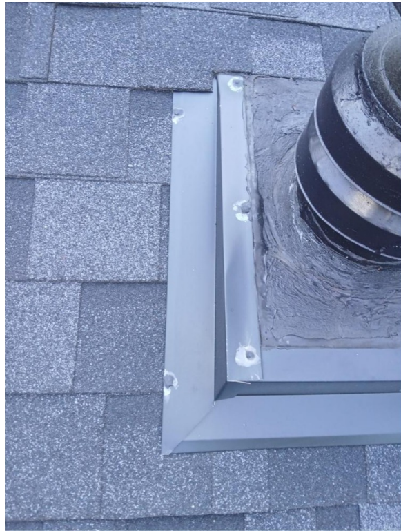
Plate 8 Second penetration, fasteners through the apron
