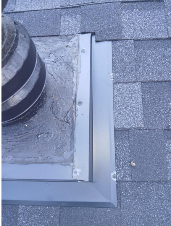
Plate 7 Second penetration on top of the shingles
